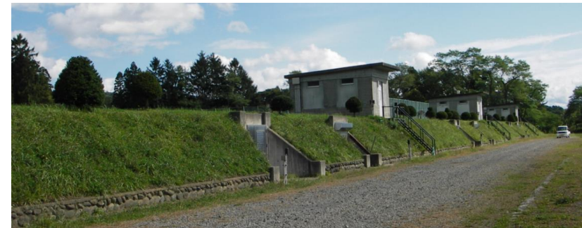
Covered filter: Otaru, Hokkaido, Japan from 1927
