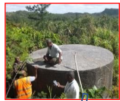
Rain harvest tank of 2.7 tons
