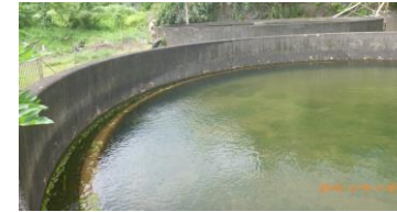
Diameter 17.8 m Area 248.8 m 2 2 tanks Retention time: 3.3 hrs
