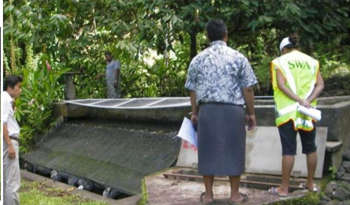
Intake Bar Screen filter
