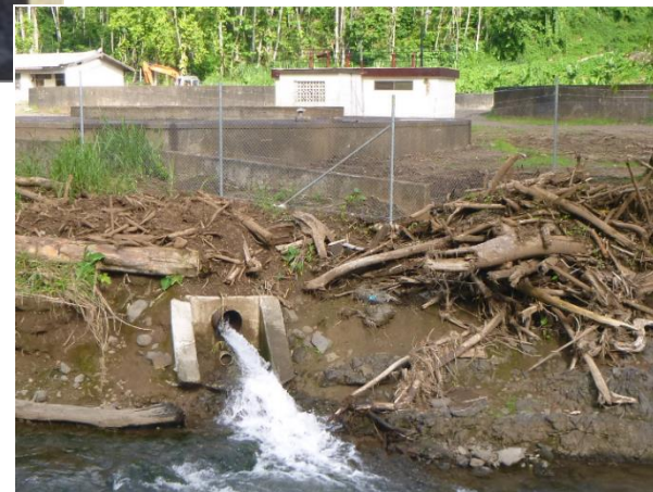
Over-flow from the balance tank for filtrate water.
