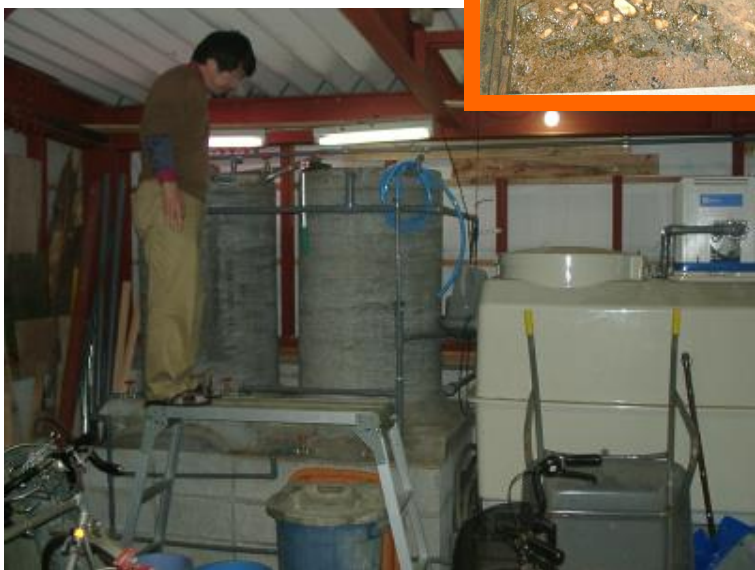
Final treatment of slow sand filter.
