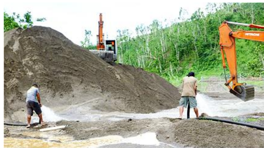
Only the sand was put on the gravel layer using a cloth to separate them.
