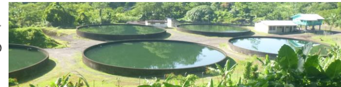
Diameter 28 m Area 616 m 2 5 filter ponds Flow rate: 3m/d
