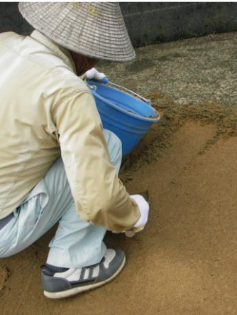
Scraping the surface at Ishigaki plant.
