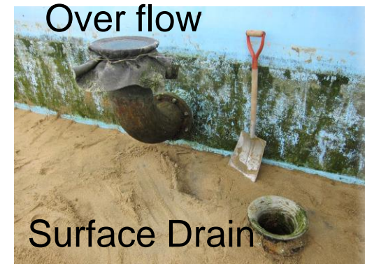
Surface Drain before scrape the surface.
