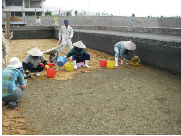
Scraping the surface at Ishigaki plant.
