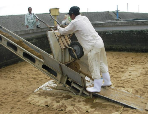
Scraping the surface at Ishigaki plant.
